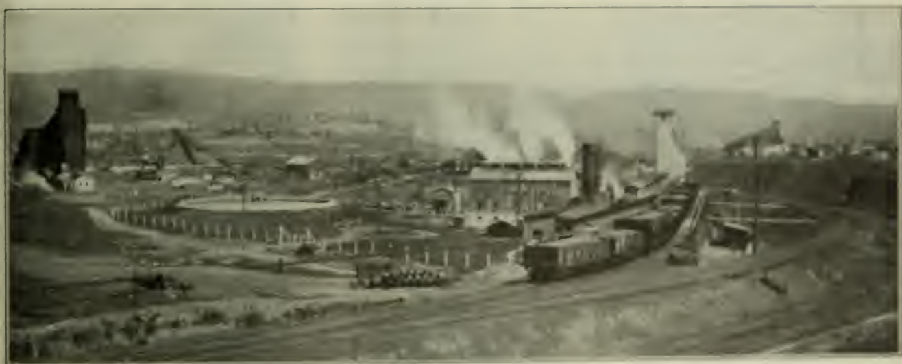
FIG. 1. GENERAL VIEW OF THE SITE OF THE HAMPTON POWER STATION.
